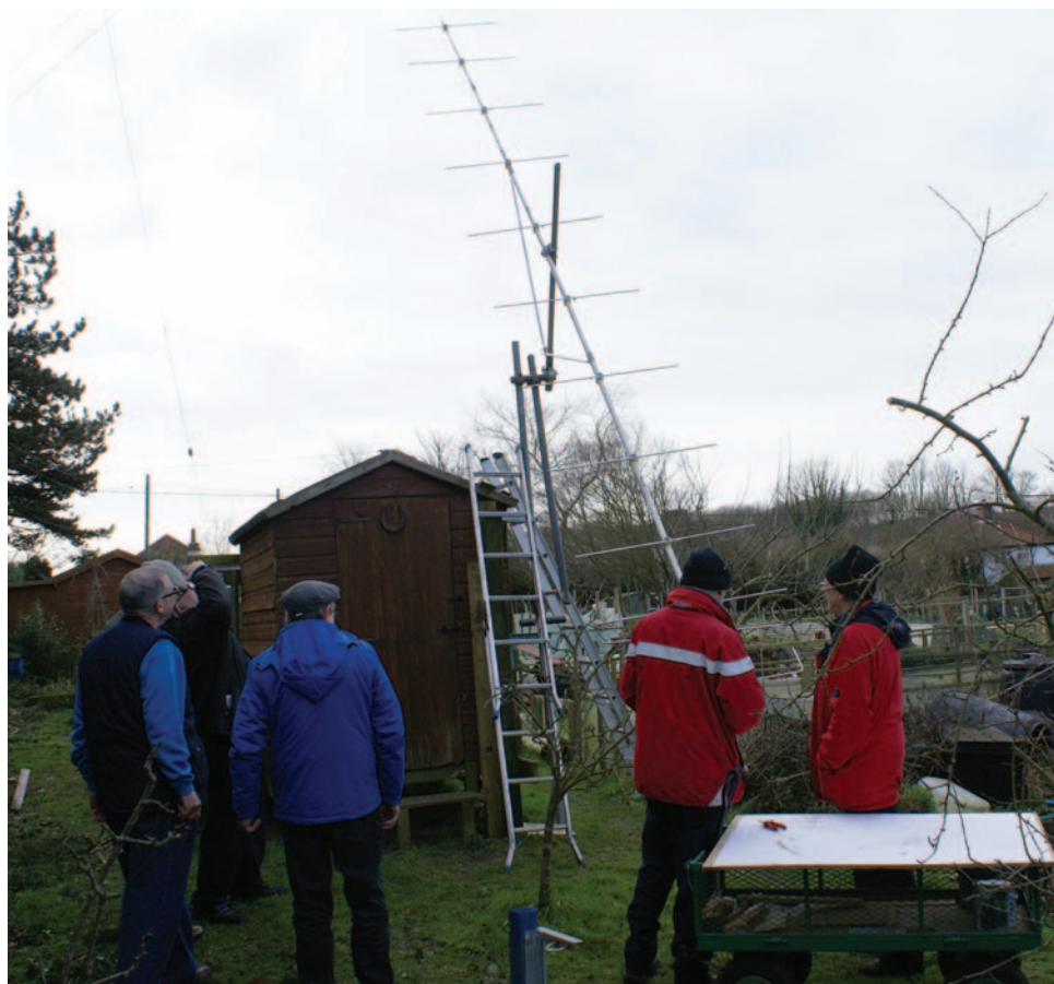
Norfolk Coast ARS has continued their experimentation with EME by constructing a 12-element 2m Yagi – on an 8m boom. Here it is shown on the simple manual pan/tilt arrangement that is located on a shed on an allotment adjoining the club's facility. The location gives a clear view of the horizon from due south to west – and now it is just a case of waiting for a Thursday when the moon is in the right position during the club's meeting.
