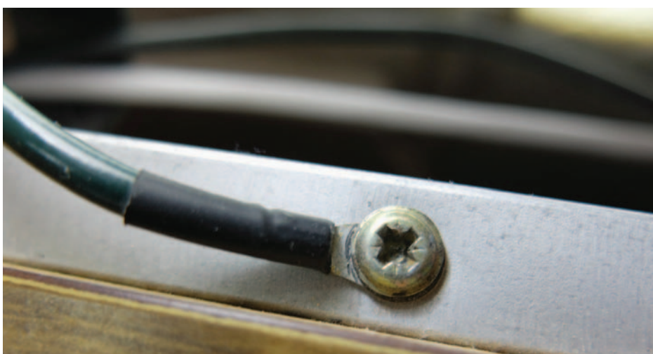
PHOTO 7: Connection made to earth bar.
