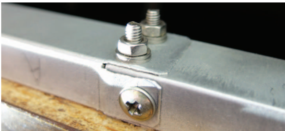
PHOTO 5: Joint between lengths of rectangular tubing.
